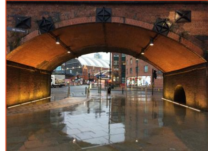
Main opened-up railway arch located on Whitworth Street South
