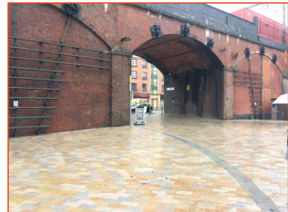
Additional opened-up railway arch located on Whitworth Street South
